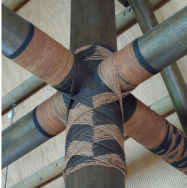
Fig. 4 Lalava covering post/beam connection [Photo: author, 2017]
