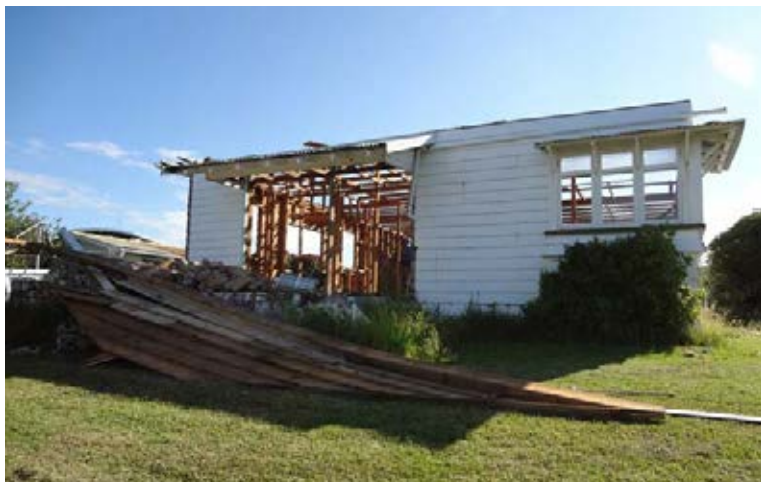
Fig. 3 The initial house being disassembled. [Photograph, Michael Davis, 2012]
